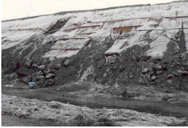
Failure of erosion-control matting.
