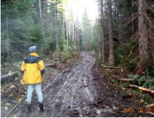
A typical access trail. Note that debris is not pushed into standing trees and is easily pulled back onto the road surface during reclamation.
