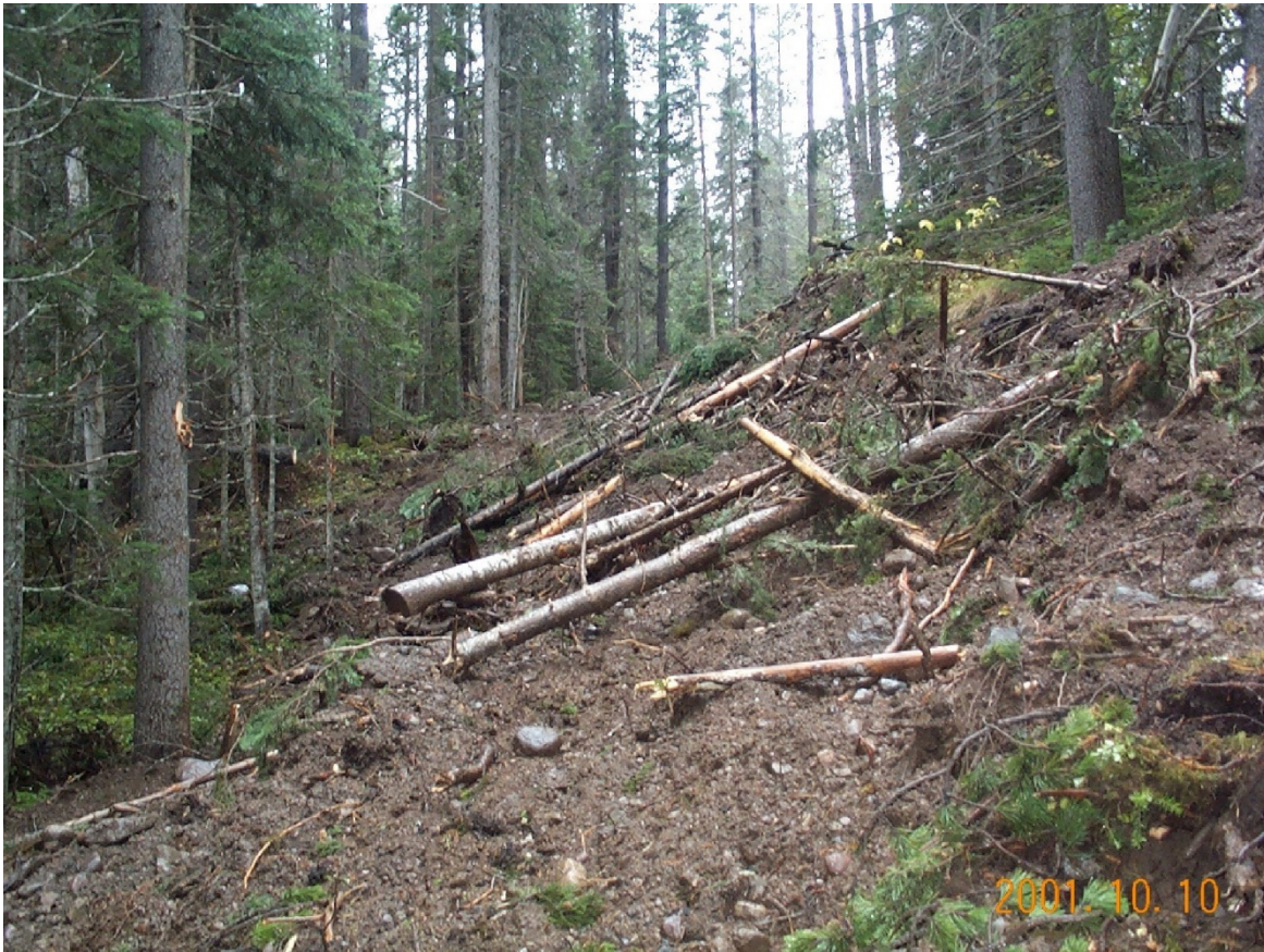
Reclaimed access trail in a moderately-steep forested slope. On slopes like this, timber and woody debris pulled over the road help to stabilize the soil before plants regrow (photo from the Handbook for Mineral and Coal Exploration in BC).
