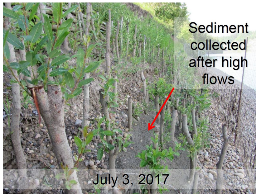
Live willow stakes on a riverbank sprout one year after planting (photo from David Polster).
