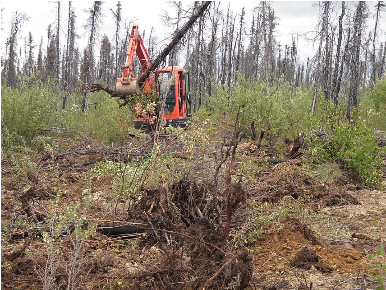
Reclamation of a trench in the Ten Mile Creek area, Yukon. Soil along with roots and stems from bushes that were removed during trenching are placed back over the trench. In addition, burnt logs and other debris from a recent forest fire were used to help reclaim the site (photo from Stewart Basin Exploration).
