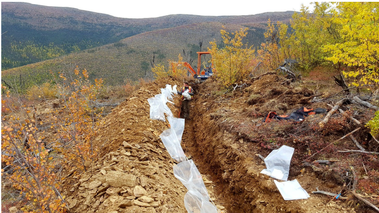
Small footprint trench in Yukon that was dug with a helicopter portable excavator. Note that the organic material has been placed on the upslope side of the trench (right side) and rock on the downslope side (left). Small portable equipment will limit ground impact and avoid the need for road building (photo from Stewart Basin Exploration).
