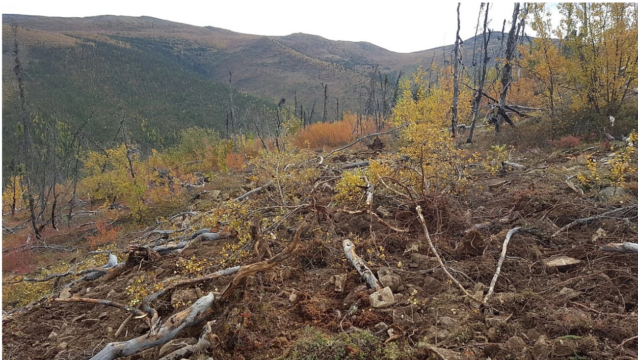
Reclaimed trench in the Dawson Range, Yukon. The ground has been recontoured to the natural slope and stabilized with woody material and bushes placed on top of the soil (photo from Stewart Basin Exploration).
