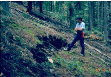
Tension cracks on steep slope.
